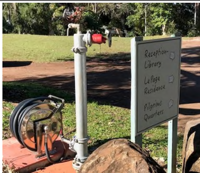
Fire reel and hydrant that the local fire brigade can connect to
