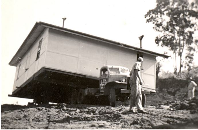
It is possible Jack Paynter took this photo. The original farmhouse is on the back of the truck ready to be driven down the slippery steep slope to its new location at Avatar's Abode in May 1958.
